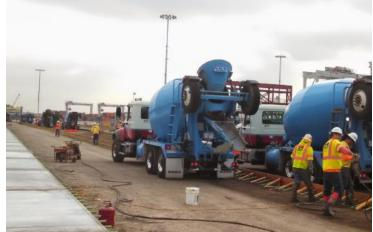
PROJECT DATA: LOCATION: Port of Los Angeles APPLICATION: Cargo Container Terminal Paving. FIBER TYPE: Tuf Strand MaxTen® CONTRACTOR: Sully-Miller Contracting Co. ENGINEER: Port of Los Angeles Engineering Division CONCRETE SUPPLIER: A & A Ready Mix TOTAL AREA: 43,000 cubic yards.
